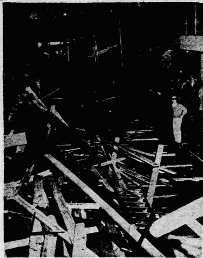
ICE SHOW STANDS COLLAPSE —An estimated 270 persons were injured 17 seriously, when the three sections of a wooden stand (above) collapsed at the Fifth Regiment Armory in Baltimore prior to the Sonja Henie ice show. The accident dropped 300 spectators 15 feet to the floor. Altogether 270 persons were taken to hospitals. All but 60 were released after receiving first aid.
