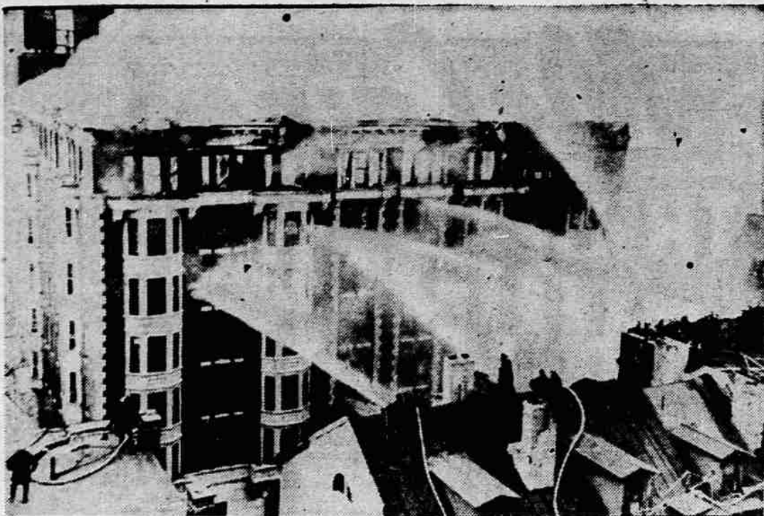
BATTLE MILLION-DOLLAR BLAZE —From adjoining rooftop, firemen battle a raging fire that is consuming the seven-story Clinton Hotel in downtown Philadelphia. The seven-alarm, million-dollar fire was the city's worst in three years. More than 150 persons were evacuated safely. Those trapped on upper floors were rescued down aerial ladders by firemen. Sixteen firemen were overcome by smoke and taken to hospitals. Fifty others were treated at the scene for smoke inhalation.
