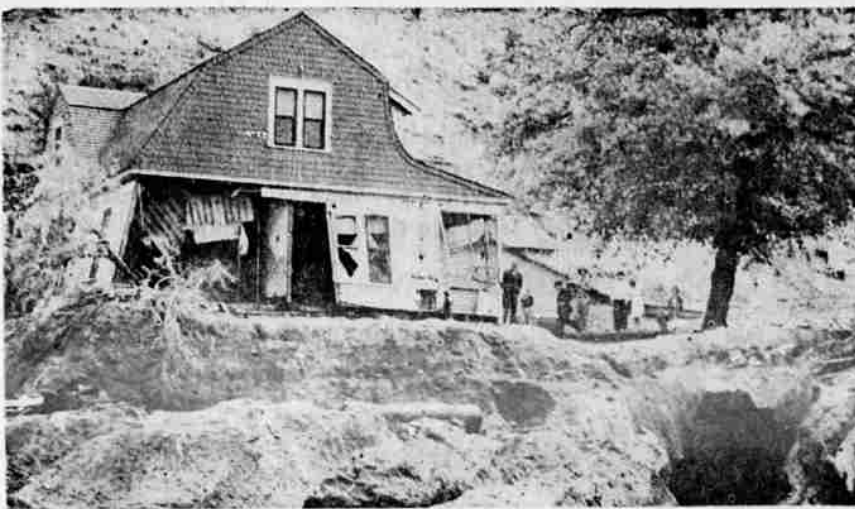
HOME DESTROYED —Farmhouse of Oscar Neibal was completely destroyed by a flash-flood that struck near Lewiston, Idaho. Neibal and his family barely reached high ground before the full force of the flood hit. Three neighbors were killed by the flood. Damage was estimated at $30,000 and 20 years of work. Note deep ravine cut by water. This was once almost level land.
