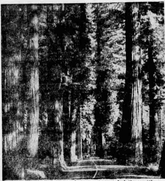
Highway is built to pass between trees, obviating cutting
