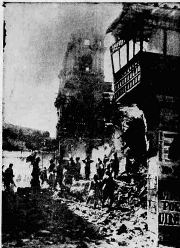
SEARCH FOR DEAD IN PERU OUAKE — Civilians and soldiers search for dead and injured in rubble-strewn street of Cuzco, Peru, ancient capital of Incas, which was 90 per cent destroyed by a disastrous earthquake. Officials have counted 56 dead and 137 injured.
