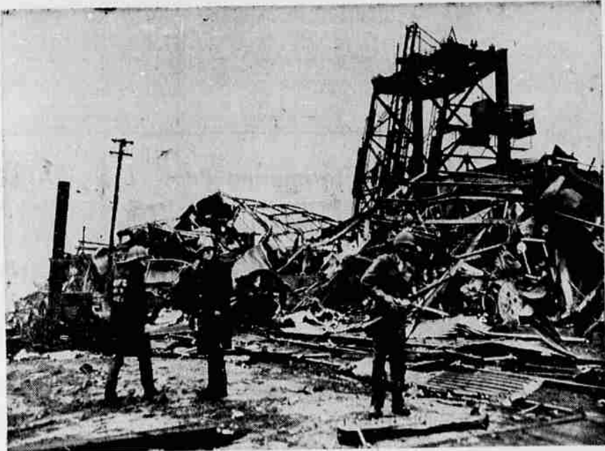
24 DIE IN PORT BLAST—Firemen and Marine guard look over debris of railroad yard near the waterfront in South Amboy, N. J., where four barges loaded with munitions exploded with a force felt in New York, 22 miles away. At least 24 were killed and an estimated 400 injured in the blast.
