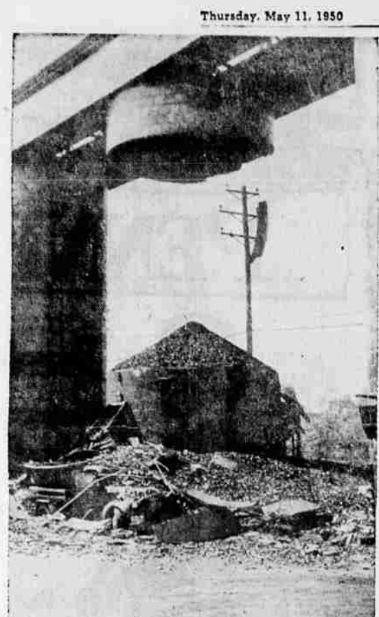
(Acme Telephoto) COLLAPSING COAL SILO Buries TWO—Buried under 100 tons of coal, two workmen in Pennsauken, N. J., escaped with minor injuries when this coal silo ruptured and collapsed. Note crushed truck.
