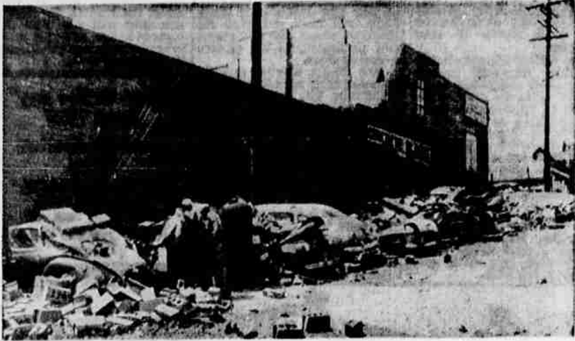
... AND THE WALL CAME TUMBLIN' DOWN—Concrete blocks litter the ground and rest on seven cars and a truck, battered and badly damaged when high winds accompanying a dust storm blew down the wall of a concrete block plant in Kansas City, Kas. The storm was the result of wild weather which left one dead and injured 88 throughout the Midwest.
