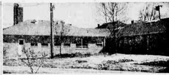
REAR VIEW —This is a view from the rear of the new Jackson county farm home near Talent. Shown is the rear or kitchen wing of the 52-bed facility that will be ready to accommodate the county's old people within a few days.
