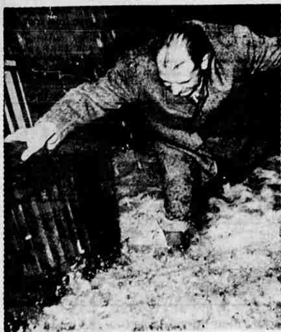
SKYSCRAPER FLOOD —Water cascades down the stairs as a New York reporter applauds his way to cover a fire on the 33rd floor of the famous 60-story Woolworth Building. The blaze caused extensive damage to offices and fixtures. The 720-foot skyscraper is the sixth tallest building in the U. S.
