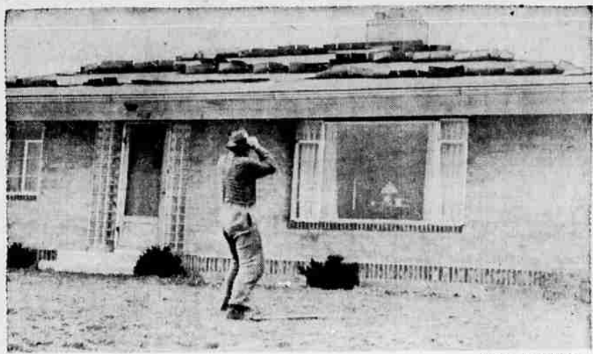
SHINGLE UPRISING—R. E. McConkey of Topeka, Kas., holds on to his hat as he watches shingles on the roof of his new home stand up and prepare to take off in the high wind which struck the Midwest. Dust storms "as bad as anything in the 30's" accompanied the winds which, at times reached hurricane velocity.
