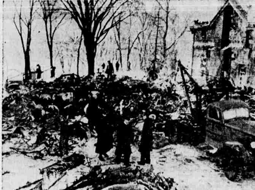
PLANE CRASH FATAL TO 15 —Firemen and rescue workers probe debris of home demolished when a Northwest Airlines passenger plane crashed into it while trying to land at Wold-Chamberlain Airfield in Minneapolis, Minn. All 13 persons aboard the plane and two children in the home died in the tragedy.
