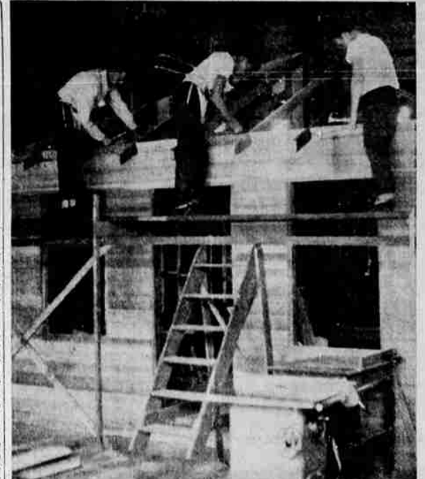
HOUSE UNDER CONSTRUCTION —The day trades class in carpentry at the high school each year builds a small four-room bungalow for actual sale on a site owned by a veteran or other qualified person. But before it is set up on the lot it is first put together in the shop at the high school as shown here. Later it is disassembled and moved to the site for final construction. All the work, including the wiring and painting, is done by the students themselves as part of the class project.
