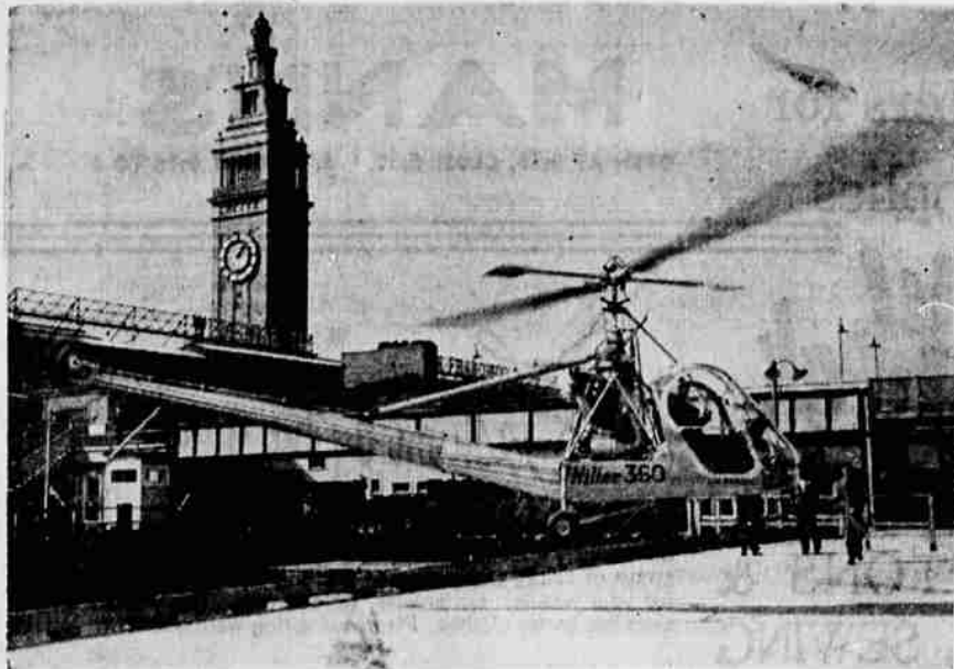
DOWNTOWN 'HELIPORT' —Helicopter hovering above this concrete island near San Francisco's famous Ferry Building will be joined by others within the next few weeks when the 5000-square-foot ramp will be opened as a "helipoint" capable of handling six to 10 helicopters at a time. The helipoint will be the only public downtown helicopter port outside New York City. It will be used for all purposes ranging from emergencies to pleasure.
