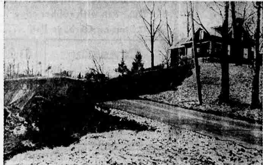
FREAKISH LANDSLIDE —Resting precariously on the edge of a huge crater, this home was almost gobbled up when an underground quicksand layer shifted in Brecksville, O. The freakish landslide wiped out 500 feet of Fitzwater rd. (foreground), warped and ruined a State Highway Department building and buckled Baltimore & Ohio railroad tracks. A family of four, asleep in the house when the slide occurred, was aroused by Water Department employees who were repairing a leaky water main nearby.
