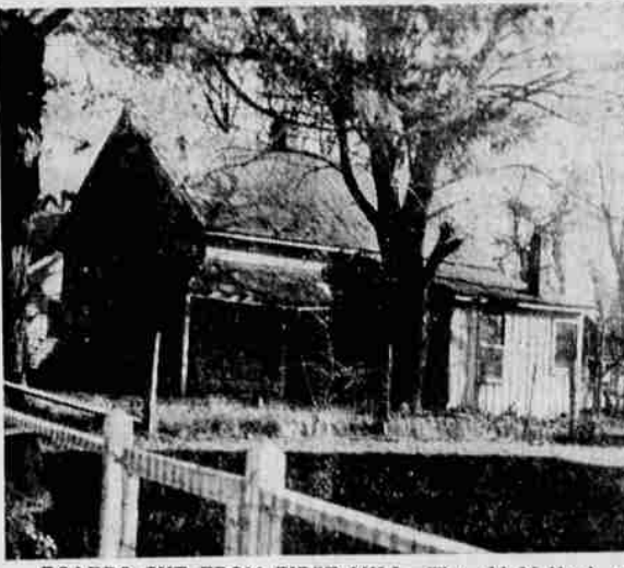
BOARDS CUT FROM FIRST MILL —The old McHugh and Herd house in Rogue River, pictured above, is one of the earliest frame houses in the community, which was originally known as Woodville. Boards for the residence are believed to have been cut by the Steckel sawmill, described in the diary of Samuel Josiah Steckel which is mentioned in the accompanying article by Elizabeth Sheffield, Rogue River.
