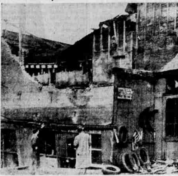
(Acme Telephoto) Worst earthquake recorded in Pacific Northwest, which rocked 120,000 square miles from Oregon north into Canada, caused this two-story, 170-foot wall of Frye & Co. meat packers, at Seattle, Wash., to topple. Damage was estimated at $30,000.
