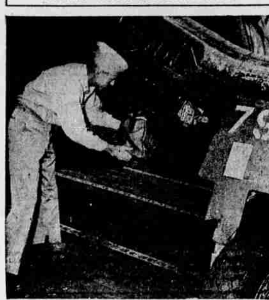
Marine Lt. Col. John F. Dobbin of Brighton, Mass., has turned a 500-pound practice bomb shell into a detachable baggage compartment on his Corsair fighter plane. The Leatherneck officer demonstrates the gadget on the flight deck of the USS Black Island, the escort carrier from which he led the first strike of a carrier-based Marine air group.
