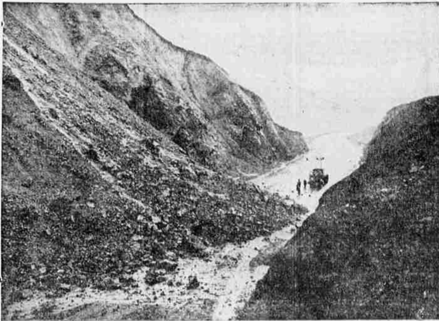
As a near record rainfall drenched California, the Weather Bureau's forecast was for continuance of "intermittent rains," which have shot the seasonal record to within an inch of the 1922 all-time high of 14.49 inches. All four lanes of the Waldo approach (above) to the Golden Gate Bridge were blocked as a result of a tremendous slide precipitated by the steady rainfall.
