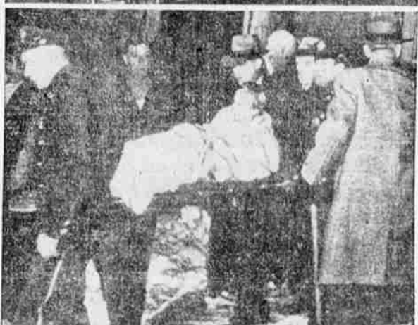
Hoses play on blazing Hartford, Conn., convalescent home where 15 died in Christmas Eve fire thought caused by defective wiring at Christmas tree lights. Fanned by strong wind, building was gutted, with only walls left standing (upper photo). One of four victims is carried from structure by rescue workers (lower photo). Four employes and many firemen were injured.
