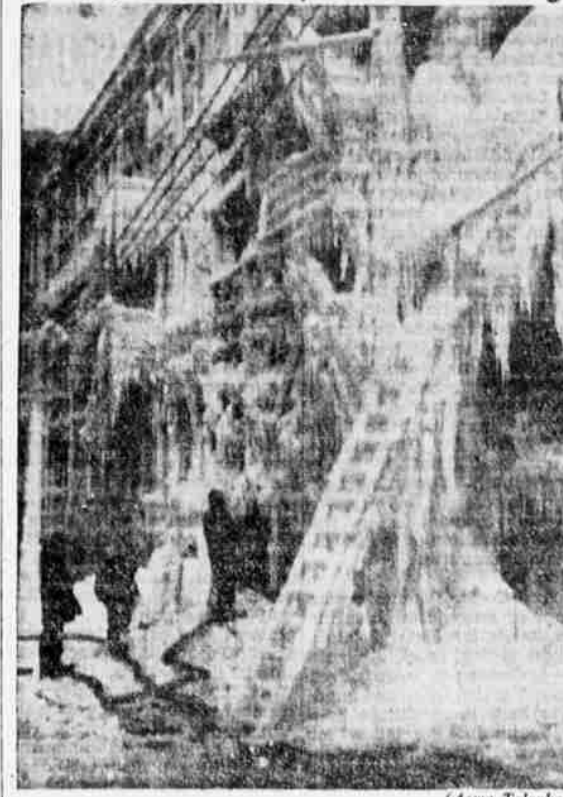
Firemen examine the ice-sheathed buildings of a business block at Akron, Ohio, following a spectacular fire which destroyed block, causing damages estimated at $500,000.
