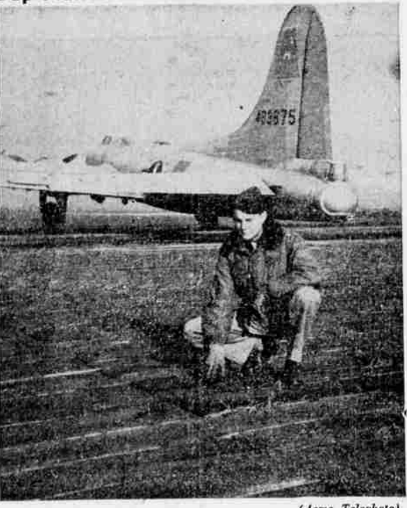
Masterpiece of makeshift is this wooden runway more than 4,000 feet long and 300 feet wide, which was used by the Japanese Air Corps at Municipal Airport, Sapporo, Hokkaido, Japan.
