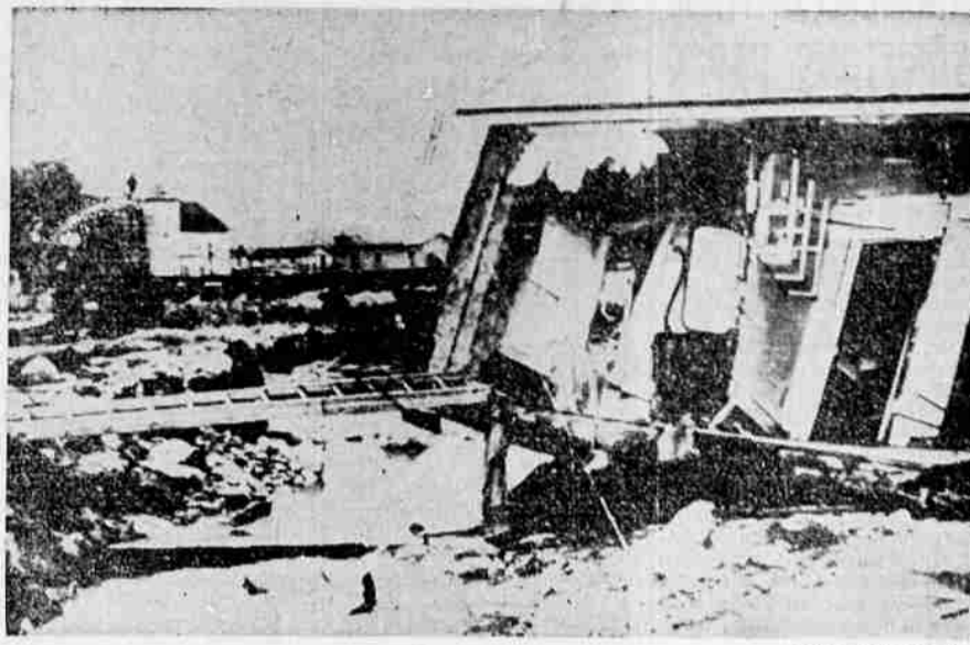
Rampaging Kinderhook Creek, swollen to river size in cloudburst, swept Steventown, N. Y., home off its foundation and washed away Rutland & Chatham Railroad bridge. Damage to highway and other property in Steventown was high and flash floods caused millions of dollars worth of damage in New York, New Jersey, Massachusetts and Pennsylvania.
