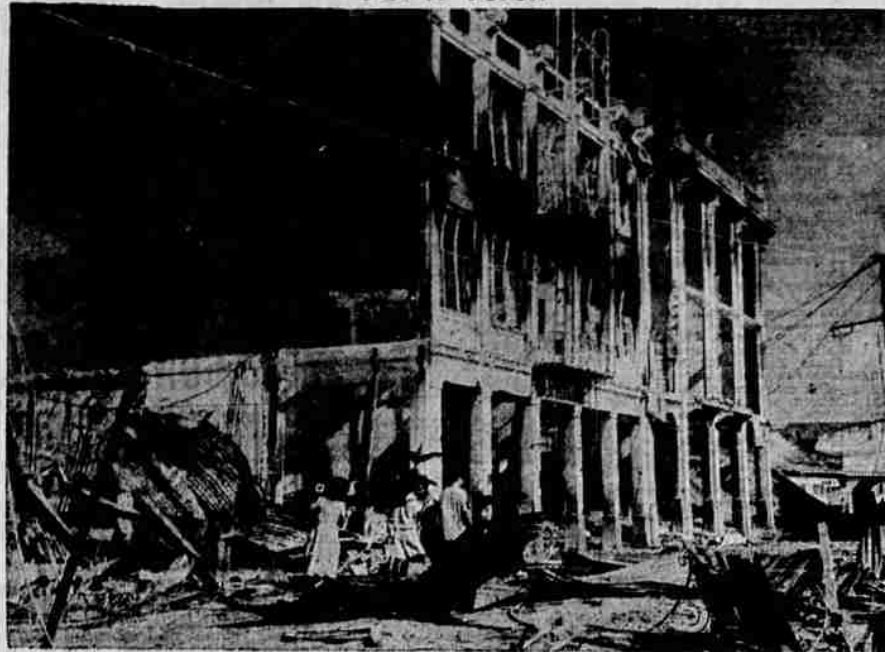
Only one wall stands of a one-time modern three-story structure on Ascaraya Street in Manila. Fire started by retreating Japs and advancing Yank artillery fire made a shambles of a large part of the city. Photo by Stanley Troutman, Acme Newspictures photographer covering the Pacific War for the War Picture Pool.
