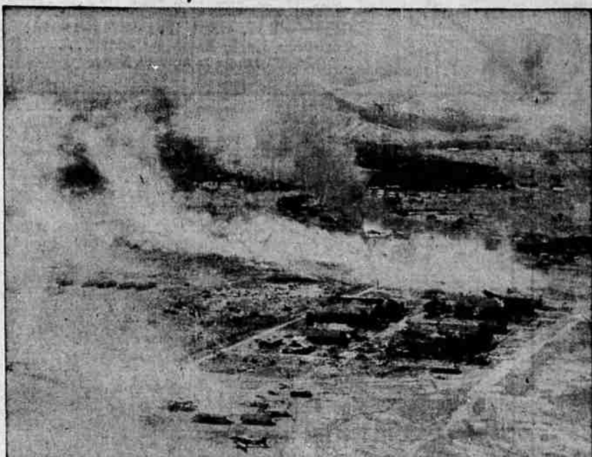
Burning, bomb-blasted hangars on Clark Field, former U. S. Philippine base, prove success of Navy airmen in their raid on the Jap-held field. The raid was made by carrier-based planes of the Third Fleet. In addition to this damage, more than 400 Jap planes were destroyed. U. S. Navy photo.
