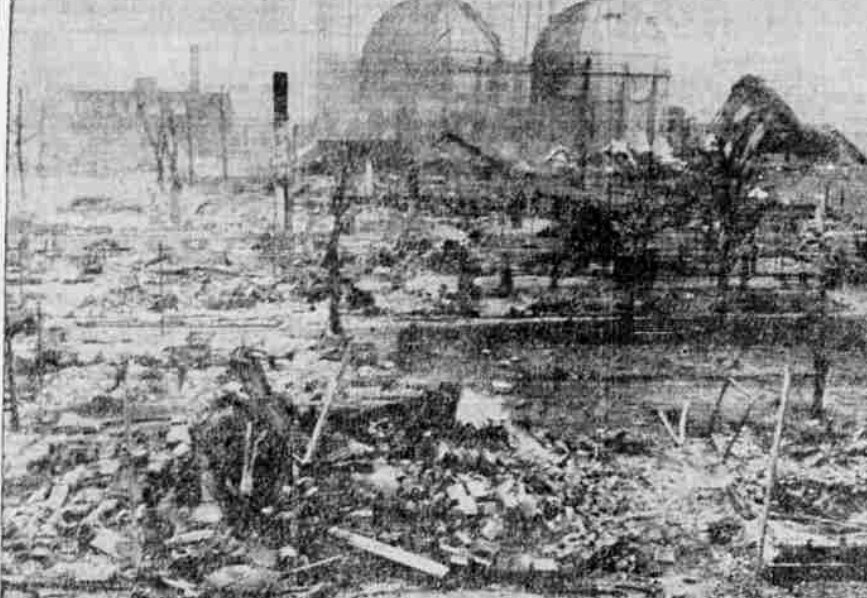
Three gas tanks stand intact amid wreckage of East Ohio Gas Co. liquid gas storage plant where thunderous explosions touched off blaze, greatest in Cleveland's history, that destroyed 50-block East Side area. The death toll will exceed 100 and more than 3000 were made homeless by the flames cascading on the heels of fiery blasts. Damage was estimated at more than $5,000,000.
