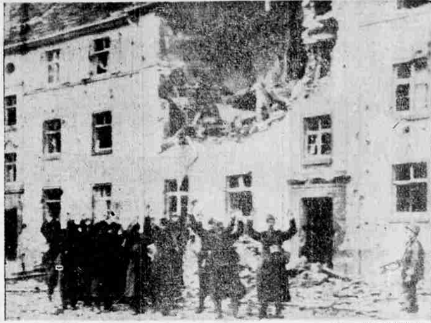
German prisoners march down street in Aachen past buildings damaged by U. S. air bombardment and artillery fire as American doughboys slugged slowly but steadily with grenades and machine guns through the street barricades of the German city. Signal Corps radio-telephoto.
