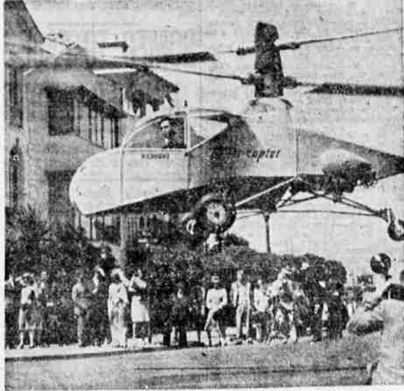
Stanley Hiller Jr., 19, of Berkeley, Calif., proudly sits at controls of his newly invented helicopter during public demonstration at San Francisco. Novelty of plane, which has attention of Army Navy officials, is construction of its contra-rotating blades which give ship both lift and forward motion. Powered by 80-horsepower motor, it has forward speed of 100 miles per hour.
