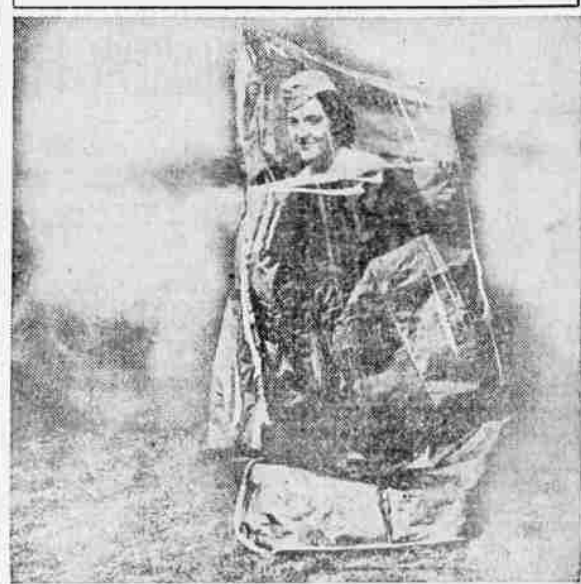
This cellophane cape, worn by Pfc. Ruth Eldon of Davenport, Ia., is a protection against chemical liquids released in battle. Designed for battlefield wear, the cape is folded into a light, compact package that service men can open and put on in five seconds flat. Used household fat salvaged by American housewives is required in the manufacture of cellophane, one of the new, indispensable products widely used in modern warfare.
