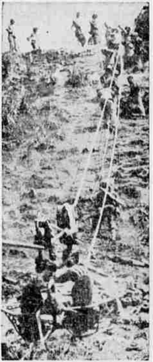
Guam's rugged terrain prevented stretcher bearers from carrying casualties down this steep cliff so they rigged up this stretcher-trolley that swiftly and comfortably lowered wounded to waiting ambulances, Marine Corps photo
