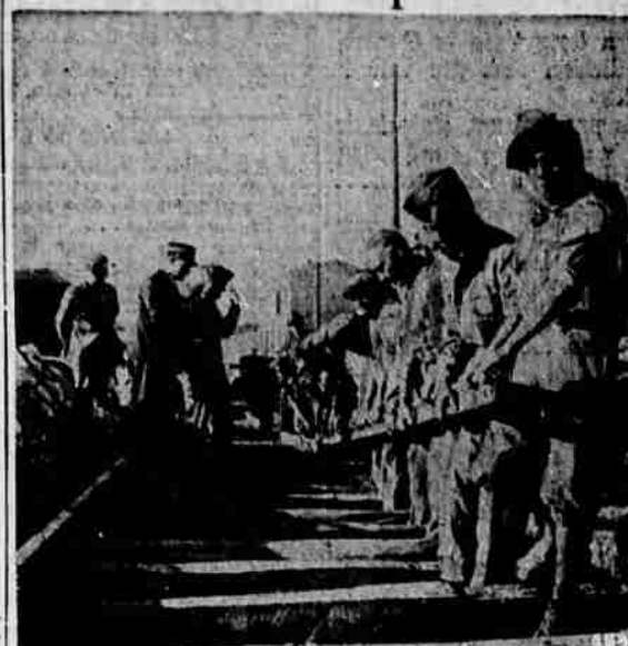
Mechanical cranes are lacking in Ternoli, Italy, so natives turn to aid British Eighth Army transport men repair railroad. Here they lift heavy rail into place. Railway was smashed by Axis' bombers before Allies took town.
