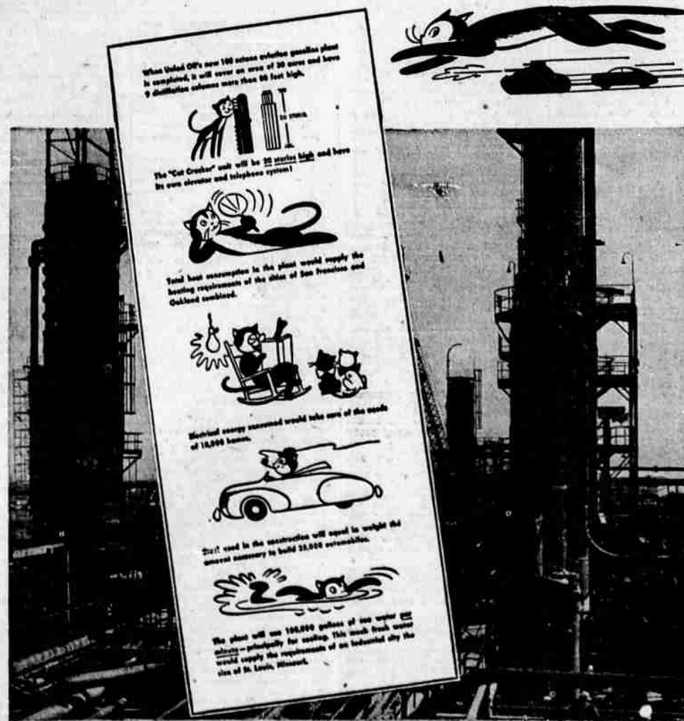
View of one section of Union Oil's new 40 million dollar 100 octane gasoline plant now under construction.
