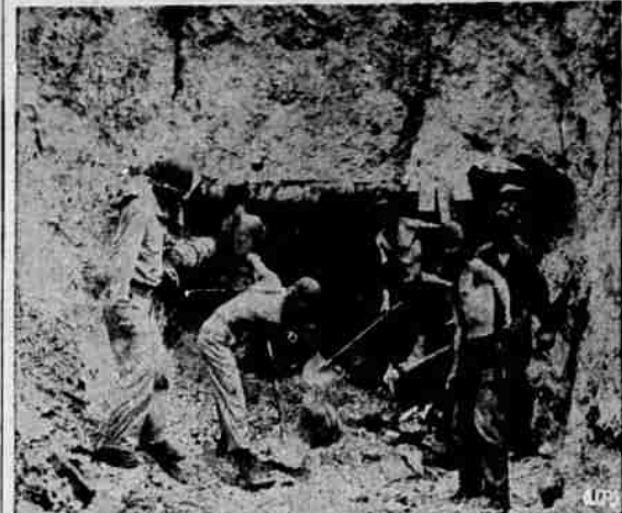
This tunnel in historic Kokengolo Hill was once an office from which the Japs directed activities at Munda Airbase. U. S. Navy Seabees are now clearing it out for Yank use.
