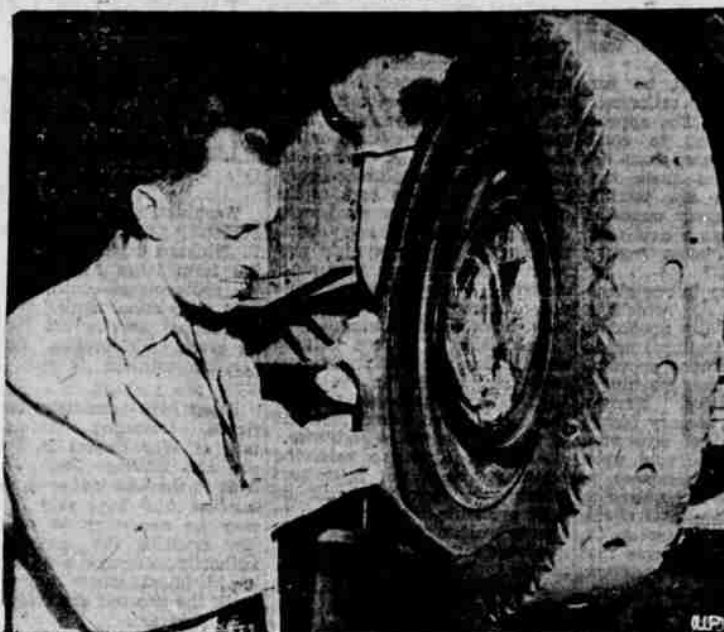
Millon Shep, Los Angeles garage owner, illustrates device for squeezing last possible bit of mileage from original tires. After cutting head from old tire carcass he fits it over the good tire, which he has deflated. Reinflates good tire and he is ready to go. Holes relieve friction heat.
