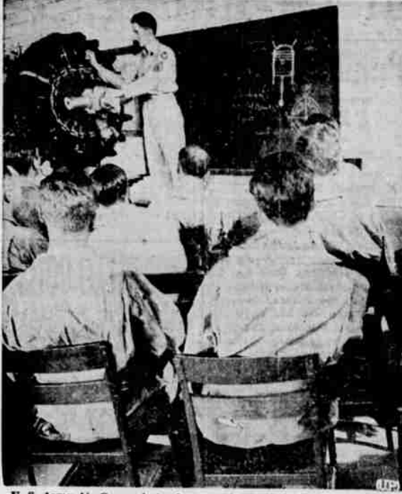
U. S. Army Air Corps photo shows mechanic-students in class listening to Sergeant Billy Eddins instructing them on valve adjustments. Innovations in educational methods have been made possible in this "on-the-job" training program.
