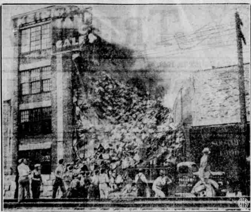
11 DIE IN CRASH —Efforts to rescue 11 workmen trapped in the collapse of a Wauwatosa, Wis., warehouse failed when part of the building crashed upon them. This striking picture was taken as thousands of beer cases avalanched onto wreckage, trapping the doomed men.
