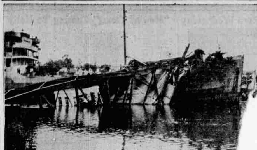
Wreckage of the 226-foot highway drawbridge over the Chesapeake and Dela at Chesapeake City, Mo., important inland waterway, lies across the bow of the which crashed into the structure. Both of the 200 foot towers on which the span fell into the canal, running between the Delaware river and Chesapeake bay.
