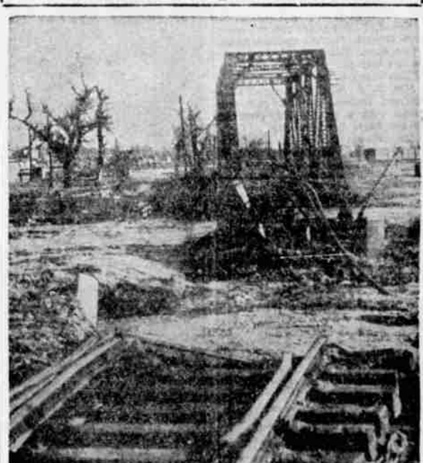
The rampaging Purgatoire river, living up to its name, tore out this railroad bridge and left Trinidad, Colo., virtually isolated. This is the main Colorado and Southern trestle; others also were washed out.
