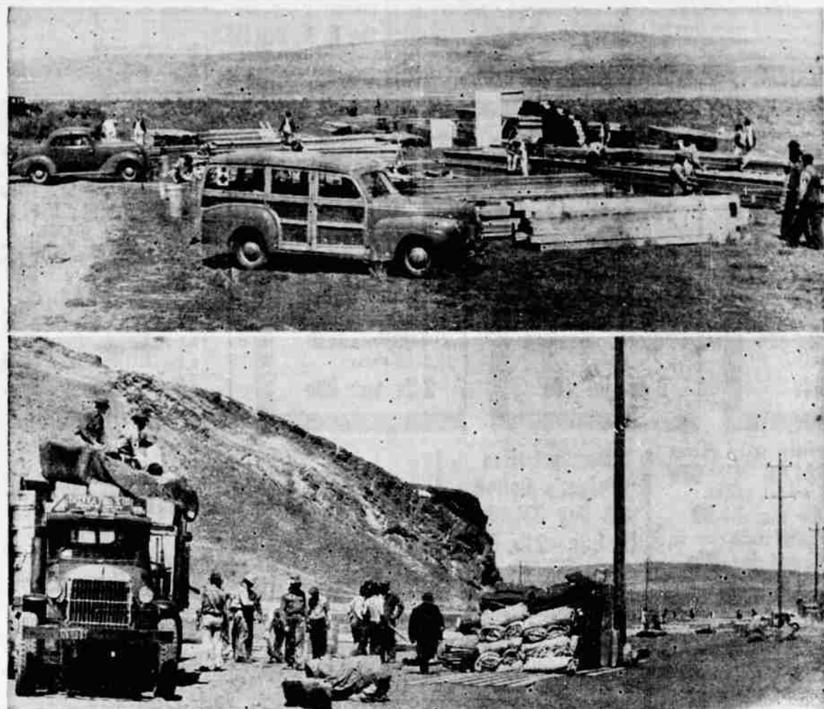
Short hours after the go-ahead signal was given for construction of the Japanese reception camp in the Tule Lake basin, workmen were on the ground laying out foundations as shown above in pictures taken about noon Sunday. The upper view shows the foundation in place for the administration building near the highway. Lower view shows workmen laying out platforms and unloading equipment at the base of the peninsula farther south.—(Photo Courtesy Evening Herald.)
