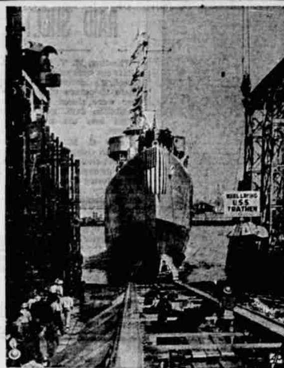
There was no time lost at the Bethlehem shipyard in San Francisco as the 1,700-ton U. S. Destroyer Frazier was launched and the keel for the U. S. S. Trathen floated into place on the same ways before the Frazier was completely in the water.
