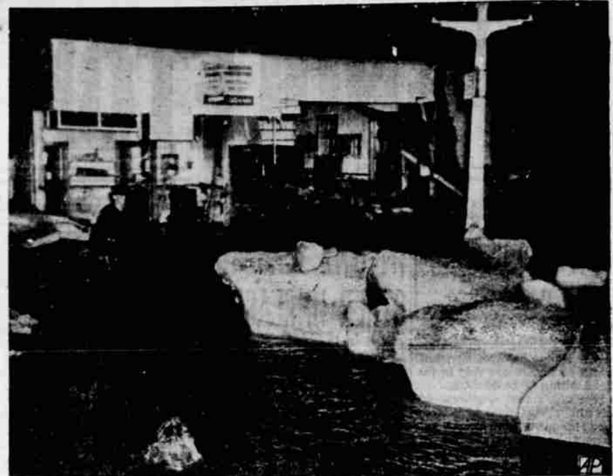
Pounding ice, carried on a flash flood due to an ice jam in the Narraguagus river wrecked a gas-line station in Cherryville, Me. The ice cakes backed into the village and two business section buildings were destroyed. Heavy rain and a thaw contributed to the high water. The jam was dynamited to release the high water.
