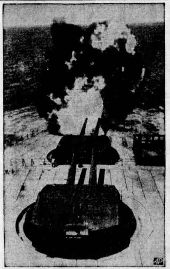
These 14-inch rifles, shown in target practice, are located on Fort Drum in Manila Bay and must be captured before the Japanese can use Manila's harbor. Fort Drum literally is a concrete battleship, built on bedrock, and is one of a series of island fortresses guarding the entrance to the bay.
