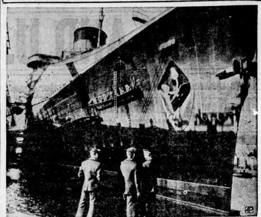
U. S. sailors watch workmen go about the job of converting the former French liner Normandie into the largest and fastest naval auxiliary in the world. The scene is at a Hudson river pier in New York.
