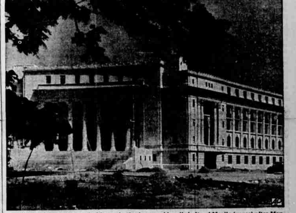
Japanese bombers wreaked havoc in the famous old walled city of Manila (upper) after Manila had been declared an open city by American officials. In the foreground is the legislative building. A direct hit was scored on the Philippine treasury building shown in lower picture which was taken recently by Deane Dickason, American author and lecturer.
