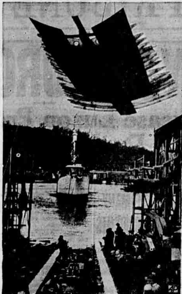
As the submarine chaser PC-485 slipped into the Harlem river at New York the keel for another one, the PC 583, was lowered into place at the Consolidated Shipbuilding Corp. yards. The navy is building the sub-chasers at a cost of about $1,000,000 each to intensify its drive against enemy submarines.
