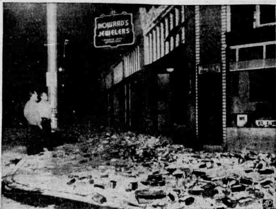
Bricks toppled from buildings in Torrance, a short distance from Los Angeles, when a sharp earthquake rocked the Los Angeles area. Bricks and glass from broken store fronts and windows littered most of this block of small stores.
