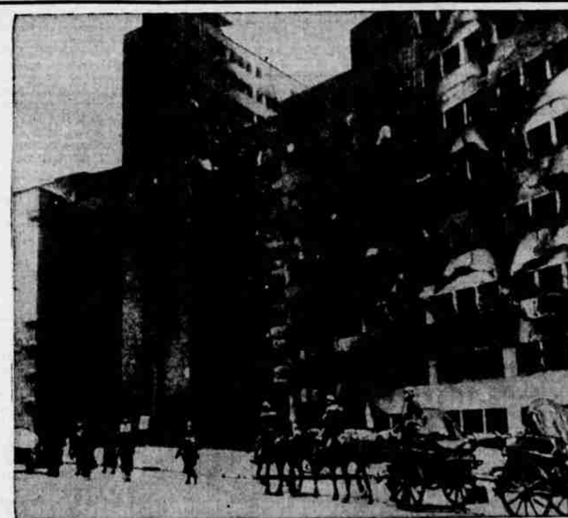
German columns pass a scorched and blackened skyscraper which houses the Soviet Electric company, in Kharkov, according to German sources. Picture radioed from Berlin to New York.
