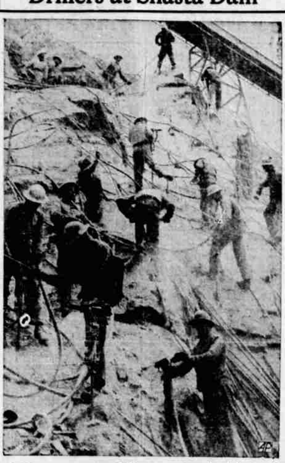
Jackhammer men are drilling more dynamite holes to blast out rock high up on the wall of the Sacramento River canyon for the west abutment of Shasta dam. They are operating drills powered by compressed air which is conveyed to all parts of the construction area by steel pipe and rubber hose from a central compressor plant.
