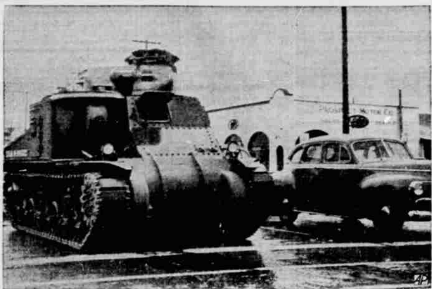
This is the first M-3 medium 30-ton tank built for the U. S. army at the Baldwin Locomotive Works, shown at Eddys Tons, Pa., on the Chester Pike headed for the Aberdeen, Md., proving grounds.
