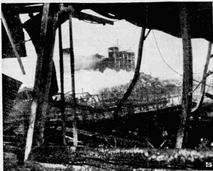
The Hudson river waterfront fire, causing damage estimated at $25,000,000, still smoldered 48 hours later. In foreground are charred beams of a Jersey City, N. J., pier-side cattle yard. Building in the background is Midtown Hudson company warehouse.
